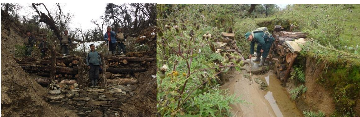
Figure 1 Checkdam construction and sediment control at Drana Gully
