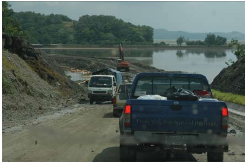
A portion of the Compact Road while under construction.
