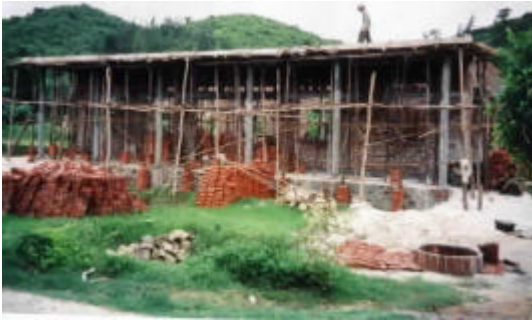
Figure 1: Building in progress
