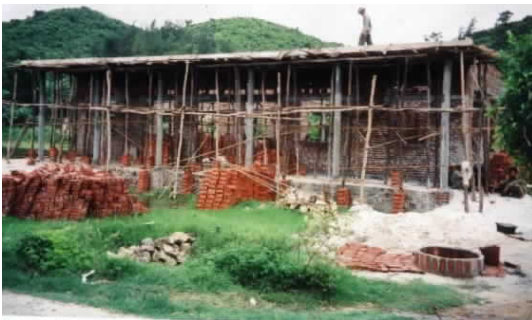
Figure 1: Building in progress
